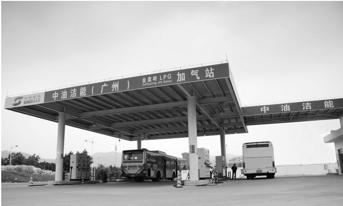
Our Jinpanling Station
